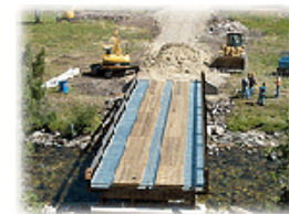
70-foot Modular Bridge Installation
