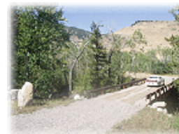
Private Ranch-owner, Modular Steel Bridge
