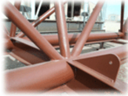
This pipe and W-beam roof truss is a very complex fabrication
