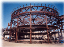
Complex Structural Being Erected
