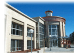
Complex Structural Completed
