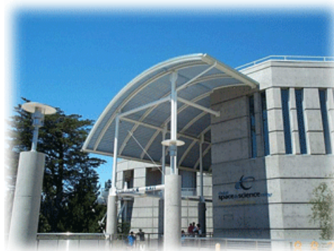
Chabot Space Center, California – Roscoe Steel Fabrication
